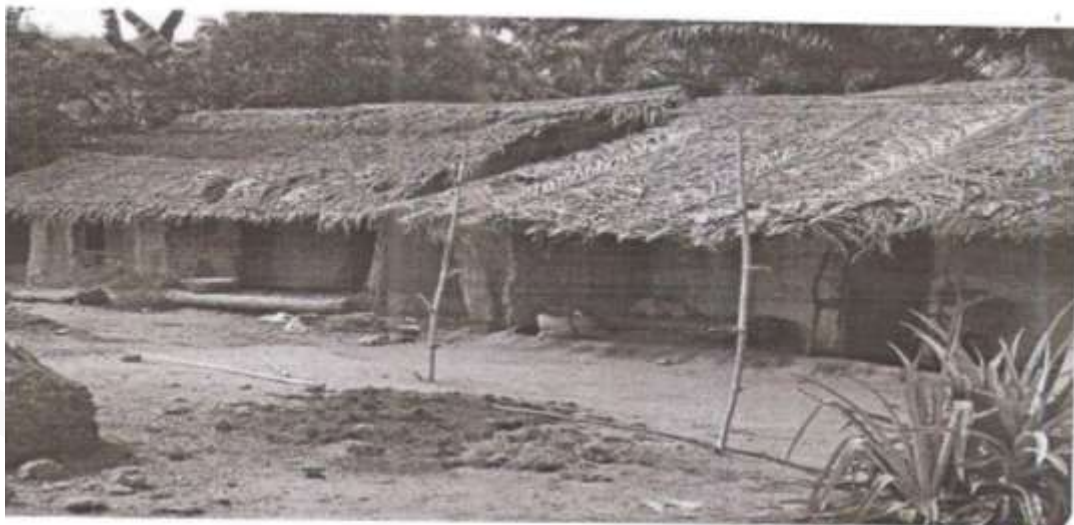
PLATE 6: THE LOW EAVE OF THE FEMALE HOUSES PROTECT THE WALLS FROM WASHING AWAY
