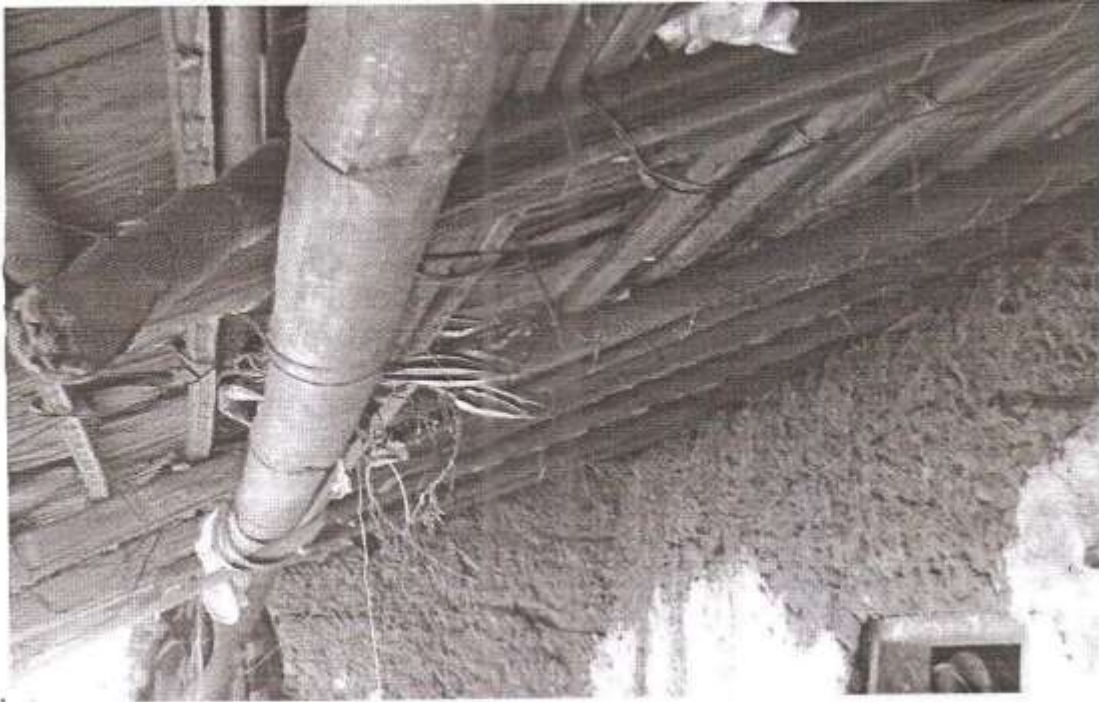
PLATE 5: THE LOW EAVE OF THE VERANDAH OF THE MALE HOUSES
